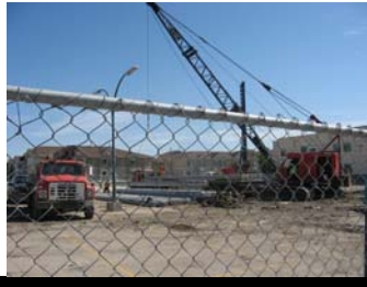
Stages of construction | July-October, 2010: construction fence installed; HQRs (high quality re-locatables) are relocated ; foundation work, including the installation of precast piles and concrete work.
